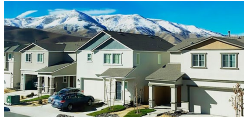
Aspen Vista at Anchor Pointe Reno, NV
